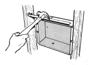
3. Extend mounting bracket, level housing, and nail to other stud.
