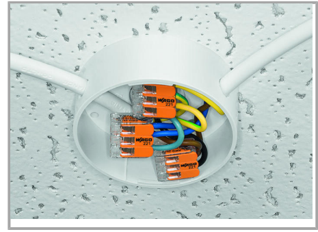
Lighting distribution in ceiling canopy
