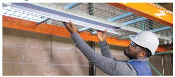
2. Cut the wire leads coming from the sockets and remove the sockets and socket bars on both ends of the fixture.
