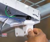
**3.** Separate mounting brackets into 3 parts. Install smaller brackets to each end, bending them over the fixture to fit the exact width and fastening them to the fixture with provided self-drilling screws. (For 8' fixtures install the wider bracket at the center of the fixture.)
