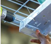
**4.** Fasten the safety cables (x2) from the retrofit pan(s) to the fixture housing using existing lances/holes of the fixture.
