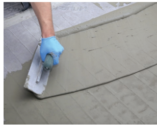
3. Trowel thinset and install flooring
