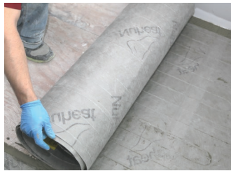
2. Roll mat onto thinset
